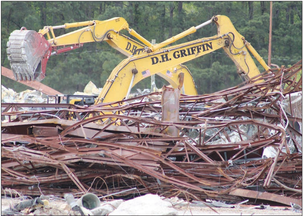
D.H. Griffin Co. excavators work near a pile of metal being recycled from the Wilson Mall in April. Drew C. Wilson | Times
