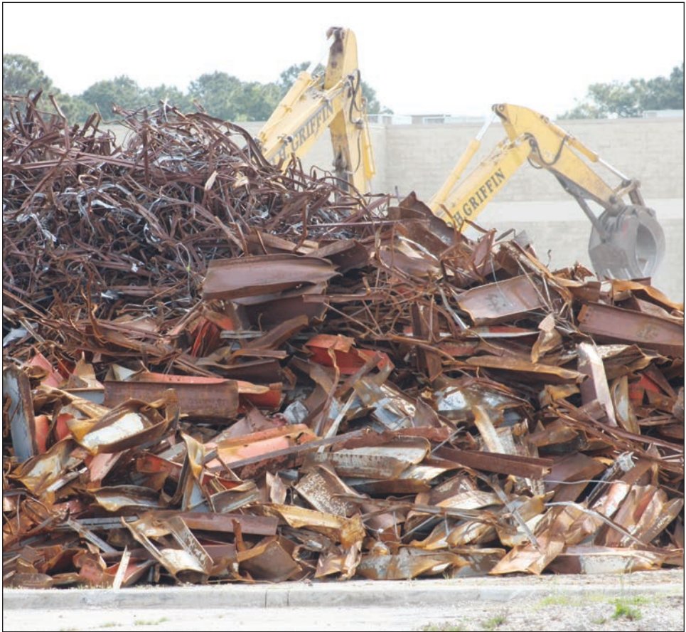
D.H. Griffin Co. excavators work near a pile of metal being recycled from the Wilson Mall in April. Some 2,425 tons of heavy steel got recycled out of the mall demo project. Drew C. Wilson | Times
