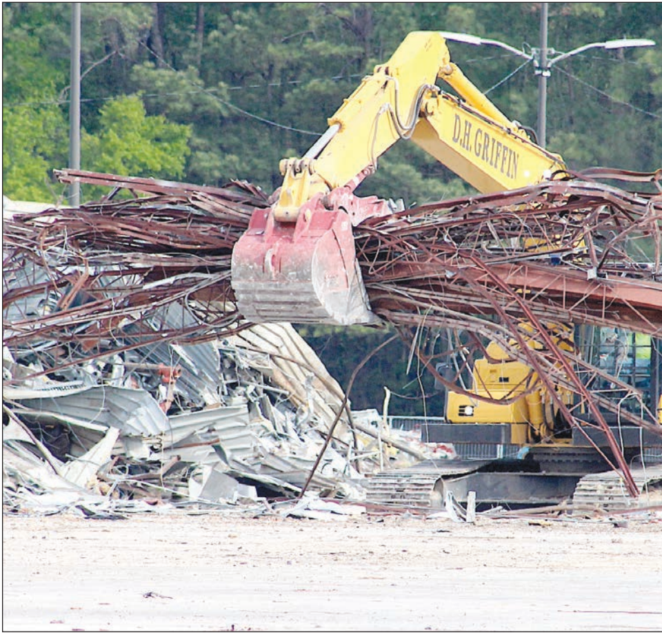
A D.H. Griffin Co. excavator claps a pile of metal being recycled from the Wilson Mall in April. Drew C. Wilson | Times
